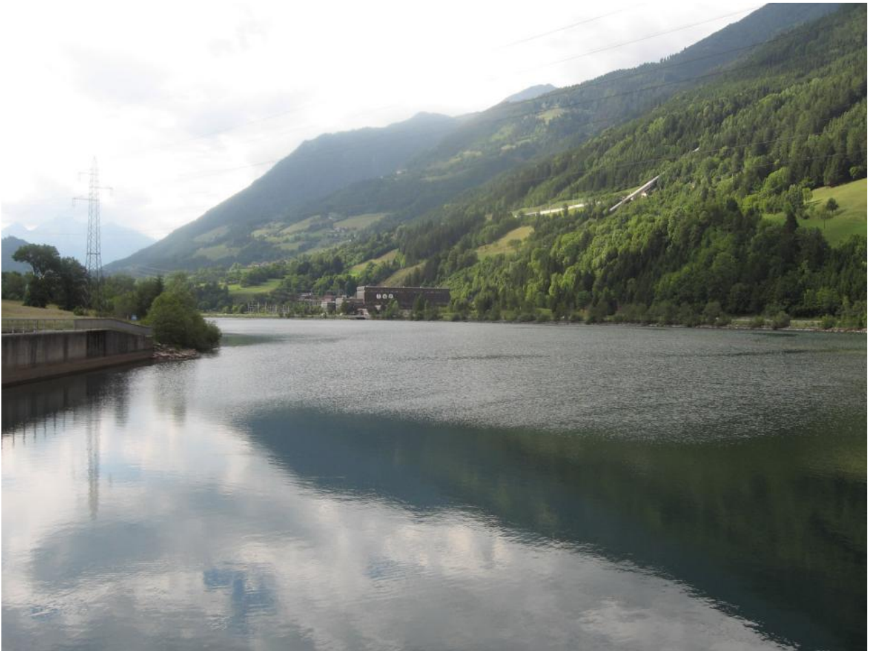
Impoundment Lake Rottau and hydropower station
