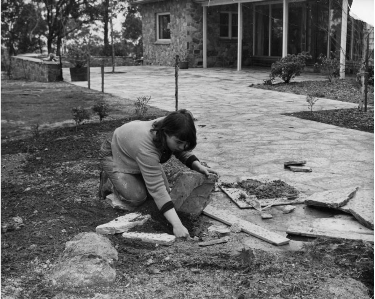
Margot Knox doing some paving (1960s)
