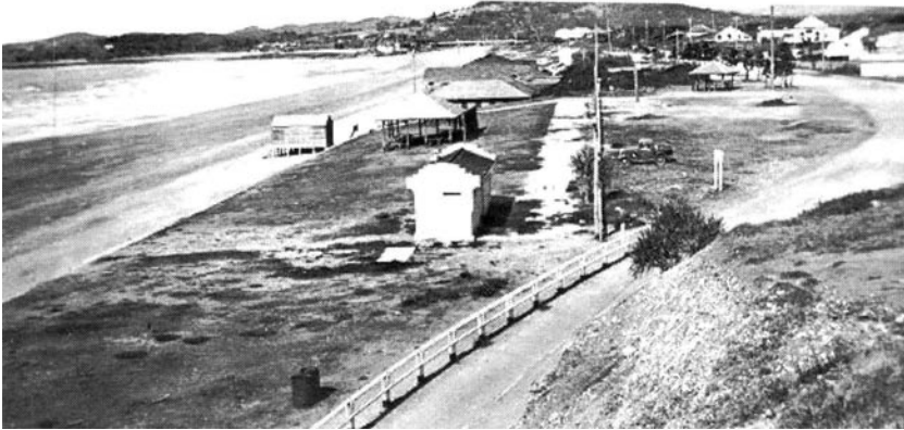
FIGURE 8. Vertical sea wall and levelled grassed area, 1938. Source: Capricornia Collection, Central Queensland University.
