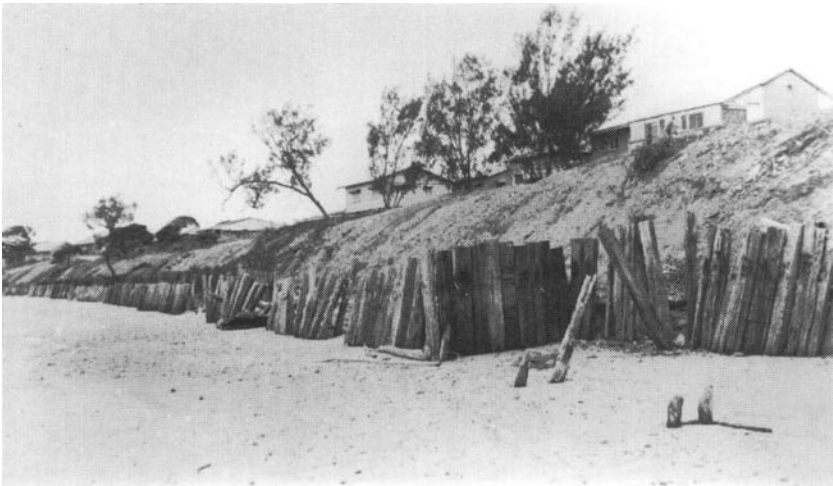
FIGURE 18. Railway sleepers vertically placed to act as a sea wall at Keppel Sands. Source: Keppel Sands Historical Society, 1995: 189.
