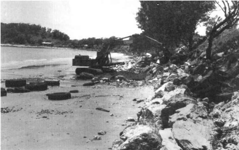
FIGURE 19. LSC constructing a rock wall on Keppel Sands beach. Source: Keppel Sands Historical Society, 1995: 85.
