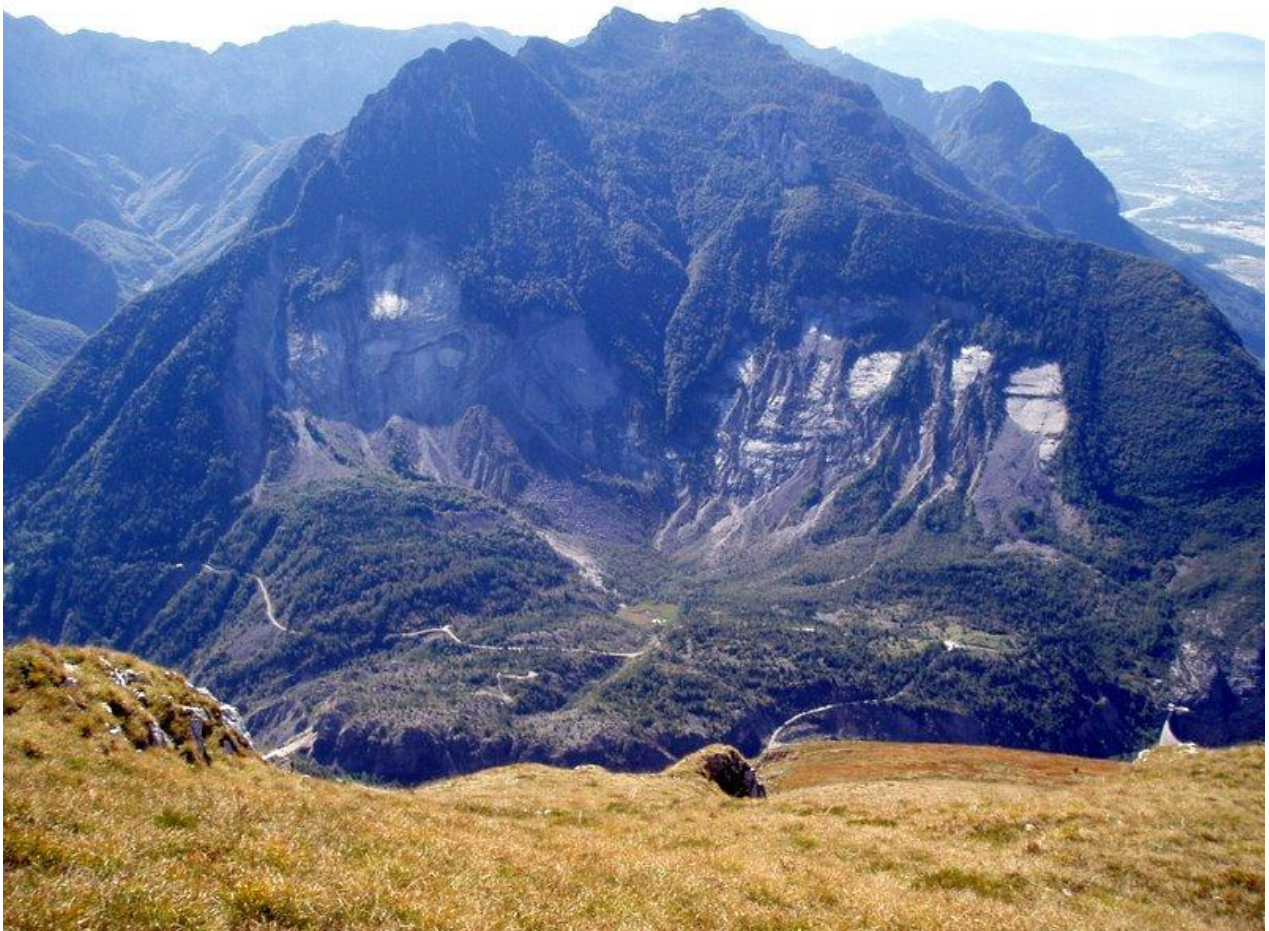
View of the detached landslide at Mount Toc.
