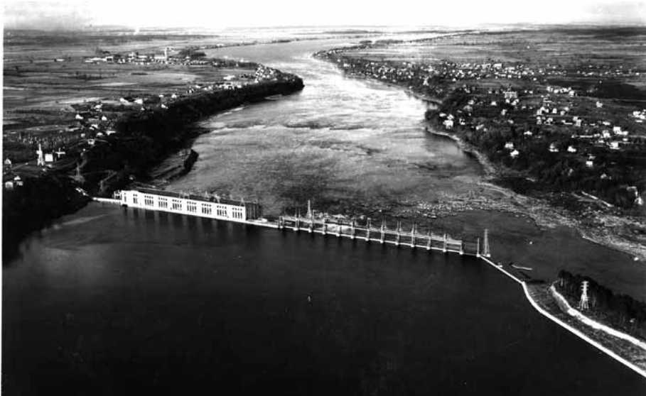
Figure 4: Hydropower plant on the Rivière-des- Prairies, n.d. Source: Archives d'Hydro-Québec H2 Commission hydroélectrique de Québec
