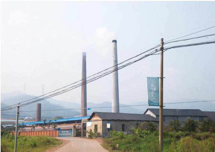
Rural coal-fired brick factory in one of China's richest provinces. (Photo: © Mette Halskov Hansen)
