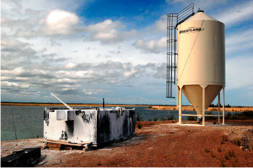
FIG. 11.2: Tailings area at the former Pine Point Mine, where overflow water is treated with lime to precipitate zinc. Photo by Arn Keeling.
