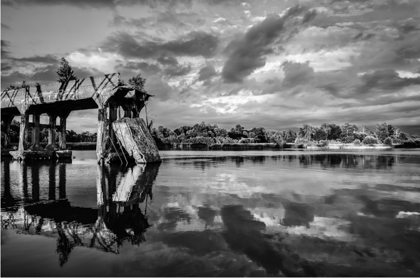
9.6 “American Ruins 1,” Escanaba, Michigan, 2011. Concrete remnants of the long-abandoned Bay Shore Road bridge (old U.S. Highway 41 over the Escanaba River). Photo by Lynne Heasley.
