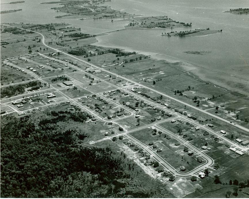
4.4 Ingleside after inundation. Reproduced with permission of Lost Villages Historical Society, Long Sault, Ontario.
