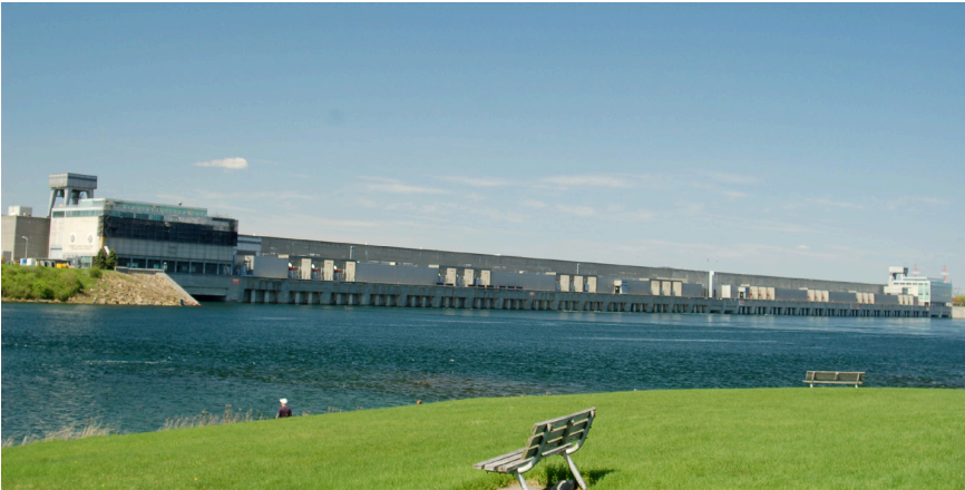
4.8 Robert Moses generating station. Photo by author.
