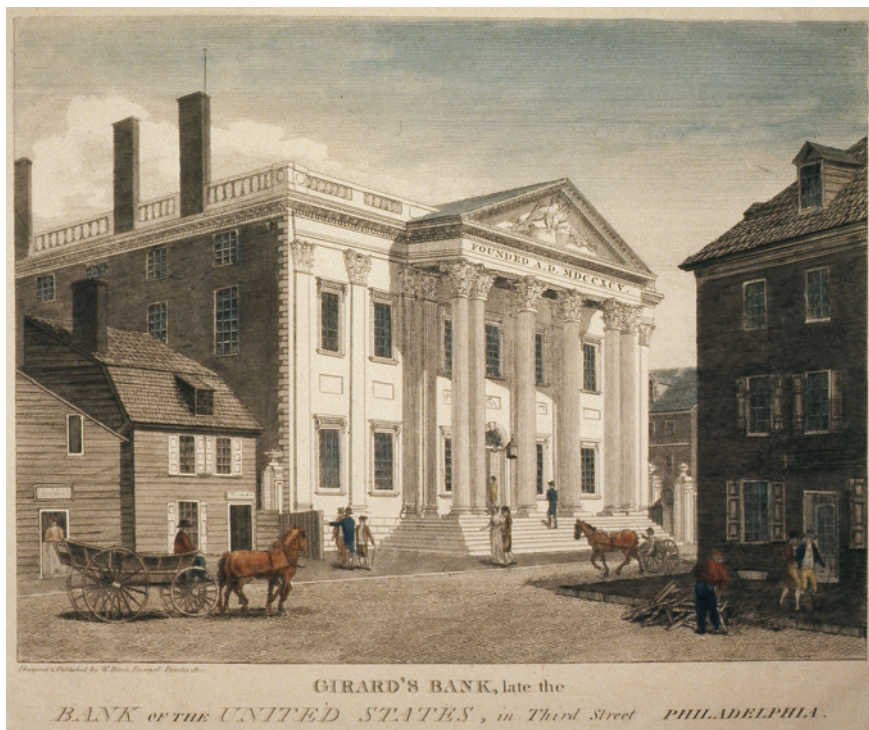
Figure 1.6. Girard's Bank, Late the Bank of the United States, in Third Street Philadelphia, plate 17 from City of Philadelphia, 1800, by William Birch, engraving, from The Library Company, Philadelphia, PA. An official seat of American finance, the bank was at the time, perhaps the most important (semi) public building in the United States and part of Philadelphia's claim on the national capital.
