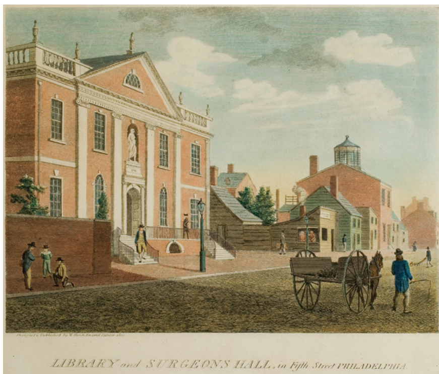
Figure 1.9. Library and Surgeon's Hall, in Fifth Street Philadelphia, plate 19 from City of Philadelphia, 1800, by William Birch, engraving, from The Library Company, Philadelphia, PA. The building, essentially a Georgian five bay house with a Palladian décor (inset statuary), exudes a feeling of balance, sobriety and dignity – an example of sturdy aristocratic republican virtue. Like Franklin's conception of the library, this is a very approachable building, a sense amplified by Birch's presentation of it. The building is tied to a street scene and includes a workman with his cart and two men who appear to be playing the gambling game 'craps' on the sidewalk.
