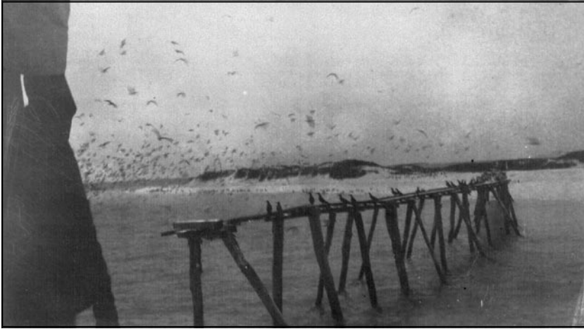
FIGURE 8. The jetty and tramline at Upolu Cay used for loading material mined from the cay, c.1933.
