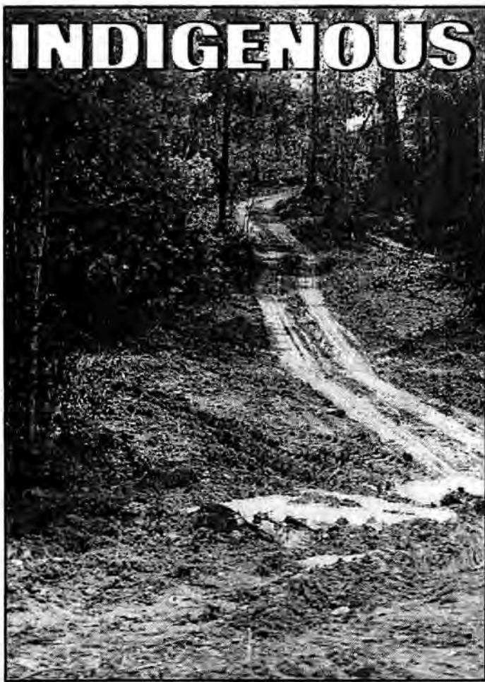
Freshly cut road paves the way for the power line
