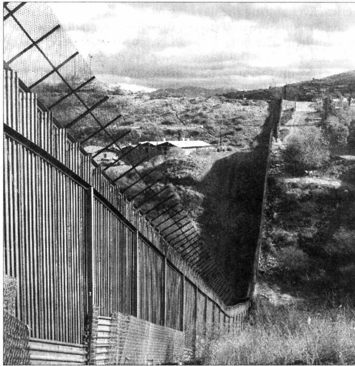
A wall made from pieces of military landing strips divides Arizona and Sonora.
