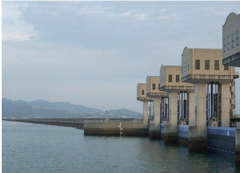
FIGURE 2. A section of the 7 km long sluice-gate across Isahaya Bay. Photo: Shigeki Imaoka
