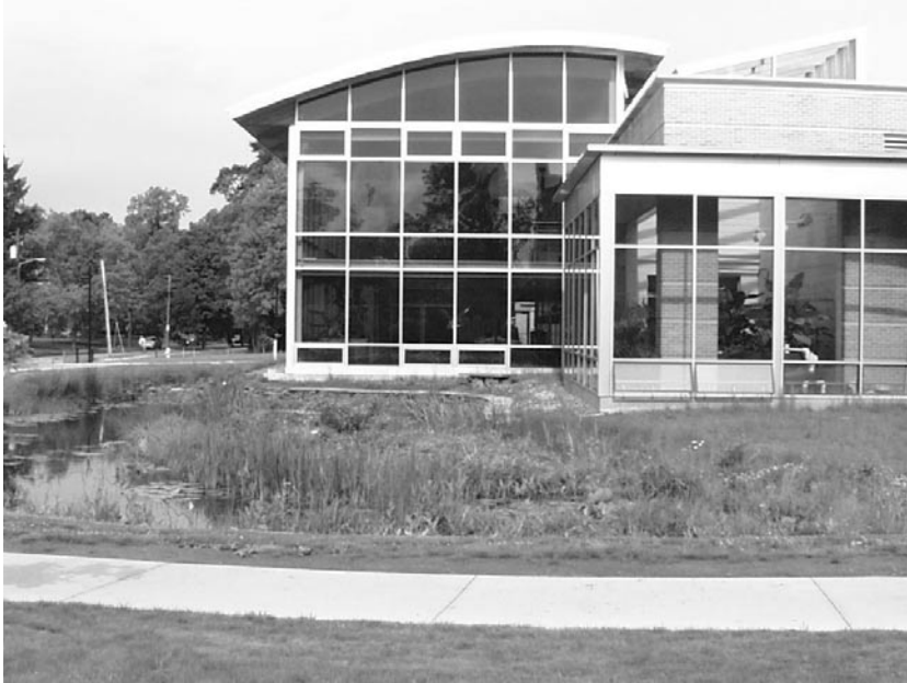
FIGURE 1. Oberlin's Environmental Studies Building and Living Machine, William McDonough, 2000.
