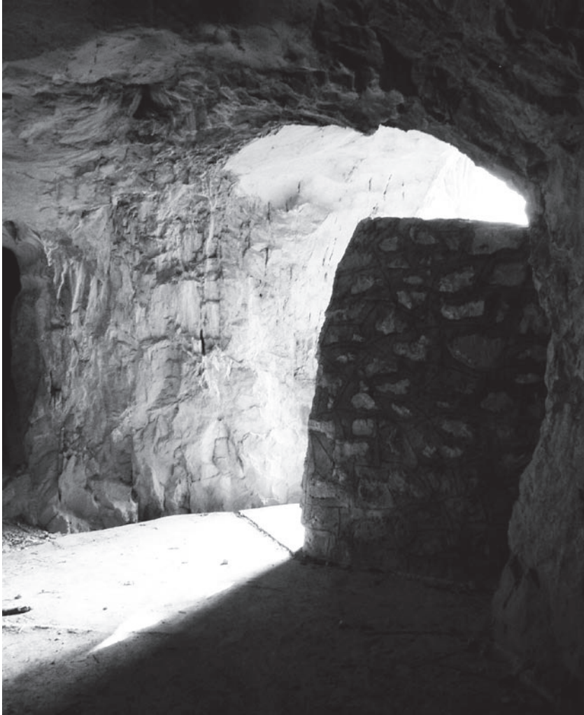
Figure 5. A blast wall constructed of stone and concrete at the mouth of a cave in Vieng Say
