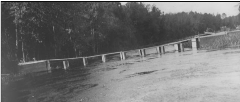
FIGURE 2. The stop-log dam in 1936. Adding or removing stop-logs between the walls or buttresses raised or lowered the water level. Photo courtesy of the National Archives, Kansas City, Missouri.
