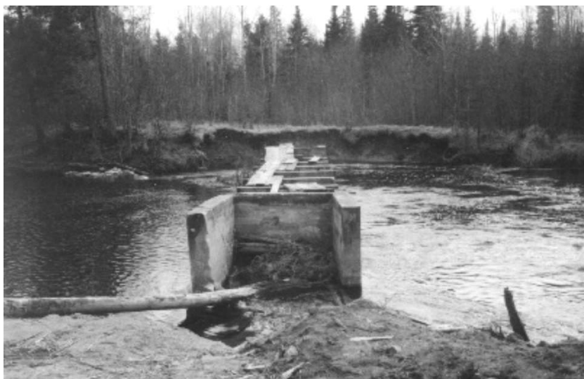
FIGURE 3. The stop-log dam in 1985. Notice the erosion on both embankments. Photo courtesy of the Minnesota Department of Natural Resources (MNDNR).
