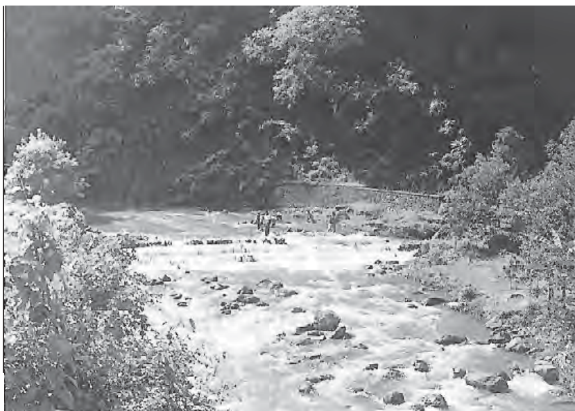
PLATE 4. The Konto river near the Tokol check dam at the end of the rainy season. Soon after the selorejo dam had been constructed, check dams and silt traps were built upstream to normalize streamflow and reduce sedimentation in the reservoir.
