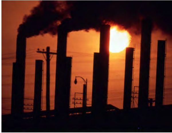
Figure 1: LeRoy Woodson: Birmingham steel plant, 10/1972 © National Archives (412-DA-11388).
