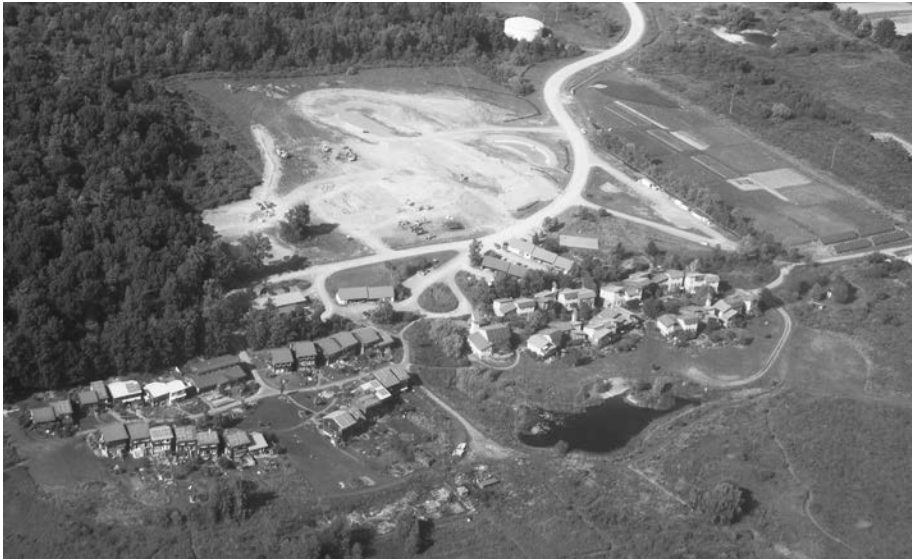
Figure 1: Aerial view of Ecovillage at Ithaca showing the layout of the first two neighborhoods and the pond. The long structures are the carpools.
