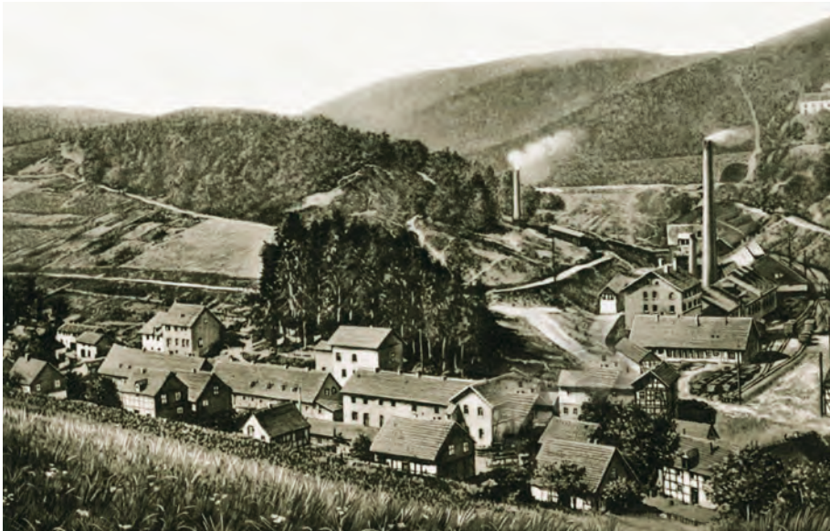
Figure 5: Picture of the south part of the Ramsbeck valley, early twentieth century. The building in the right half is the part of the smelting works of Ramsbeck where the ore was roasted (“Rösthütte”). As the picture shows, the smelting works had a high chimney, too. The smoke exhaust duct from the “Rösthütte” to the mountain on the right side can’t be seen in this picture; however, it appears in the left part of figure 2 (Source: Chronik der Familie J. Cosack , 1913)
