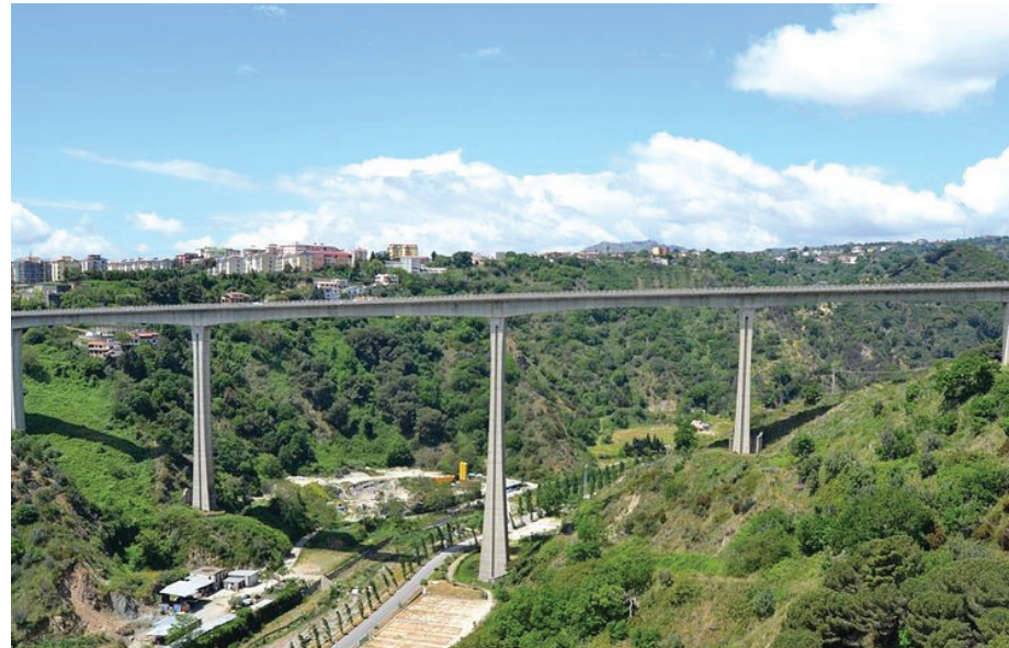
Figure 1 The Fiumarella Viaduct (Viadotto Fumarella) in the province of Catanzaro, 2013. One of the many bridges built in the uplands of Sila in order to connect different zones otherwise hardly reachable. (Source: Wikipedia, CC BY SA 3.0)
