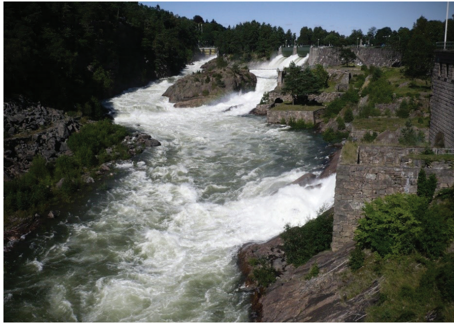
Figure 2 Trollhättan power plant and waterfall, Western Sweden, 2015 (Source: Author)
